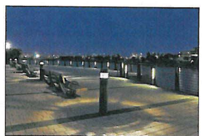
Lighting for the 5th Street Overlook remained low level so as not to obscure the waterfront view of the Mission Bay Development to the south. Custom fluorescent staplelight fixtures integrated into the handrail design and lowered bollards provide pools of light that intermingle playfully on the overlook. Photo courtesy of Marcia Lieberman
