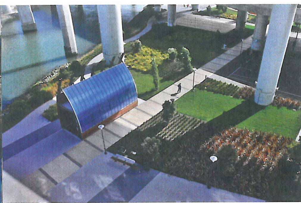
LEFT: A rich and colorful landscape weaves in and out of Mission Creek Park North expressing wave like patterns and a playful reflection of the sculptural ramps above. Dynamic and colorful during the daytime and nighttime, the kayak storage building conveys more of the park's nautical and playful theme. PHOTO COURTESY OF MARCIA LIEBERMAN
